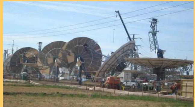
A: They are Tessera Solar's 1.5 MW Dish Stirling solar farm. The mirrors concentrate the sun's energy onto a Stirling heat engine which in turn powers an electric generator. There will be 60 dish/engine units at the site when it is completed early next year.
