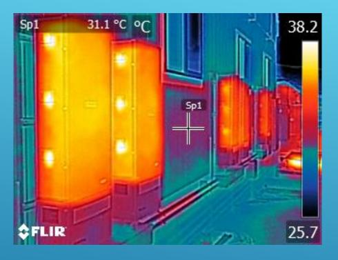
COMBINER BOXES AND INVERTERS – ARE THE STRINGS TORQUED PROPERLY ARE THE INVERTERS VENTING PROPERLY OR ARE THEY WORKING AT ALL?
