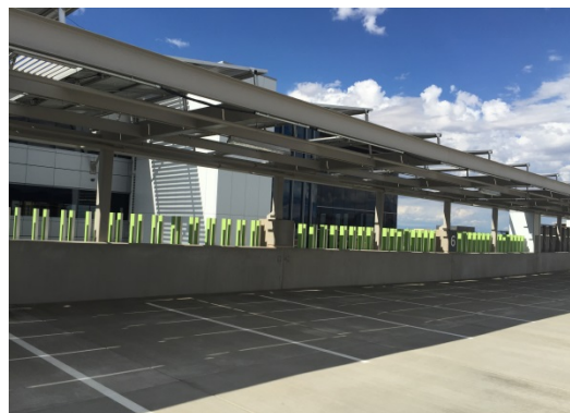
Solar PV parking shade canopy at top level of garage.
