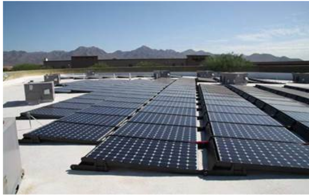
Solar PV rooftop installation below roof parapet.
