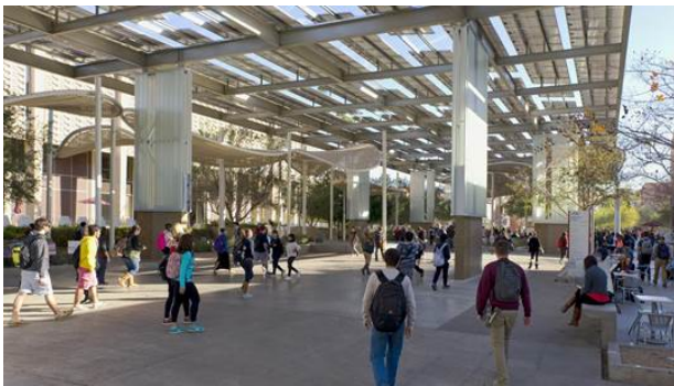
Pedestrian solar PV shade canopy.
