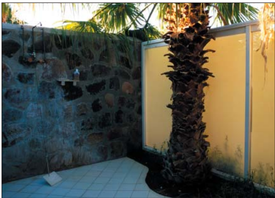
The base camp was designed to minimize use of energy and water. An open-air shower, shown here, is controlled by a foot pedal, and greywater from the shower drains directly to trees and other vegetation. Photo: Taylor Galyean
