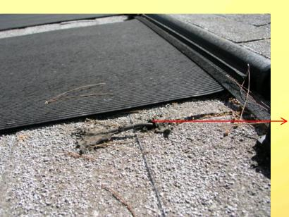
Sensor not installed correctly floating, note roof needs to be replaced
