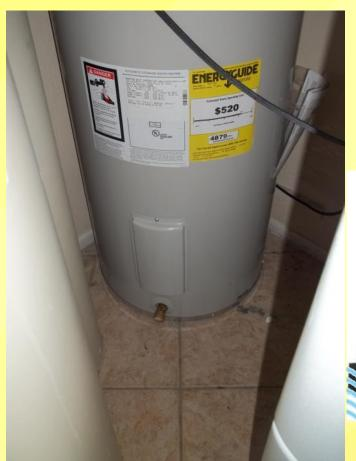
Water tanks in or above a conditioned space shall have a drip pan with a drain line to a safe location
