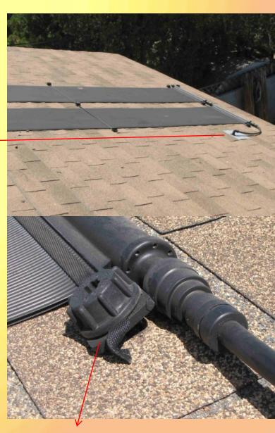
Tie-down tearing out of roof
