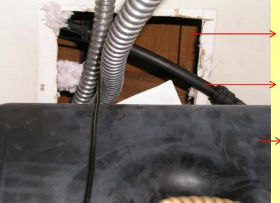
Open hole into attic, insulation falling into house
